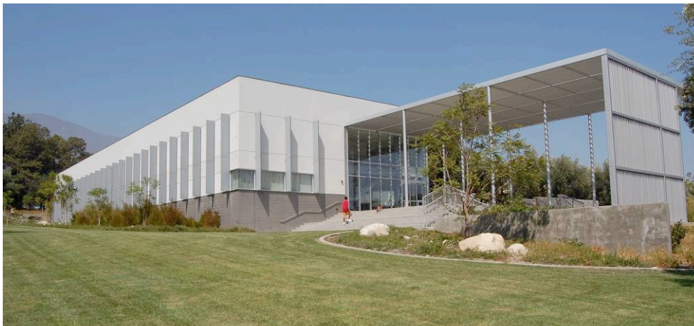
Chaffey Community College Student Services and Administration building.
