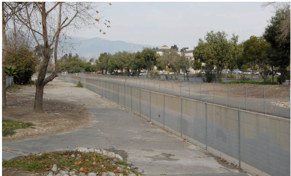
Storm drainage channel facility.
