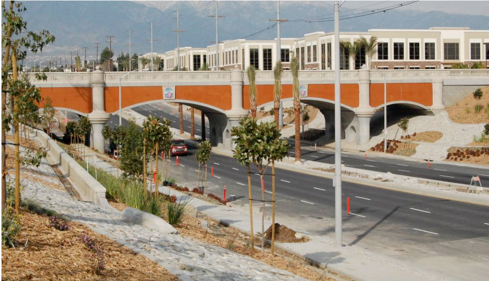
The new Haven Avenue/ Metrolink Railroad bridge: vision to reality.
