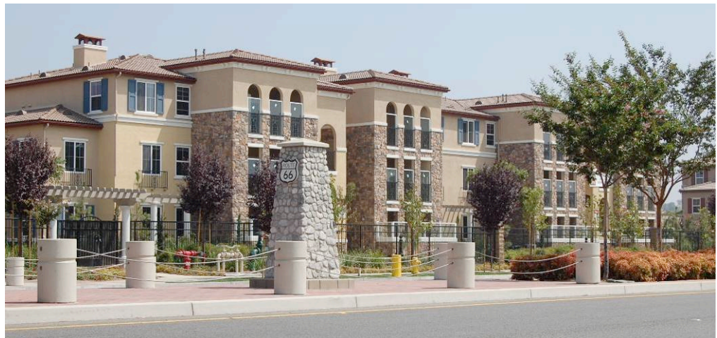
Medium High Residential Development along Foothill Boulevard between Hermosa and Center Avenues.
