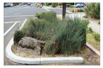
Corner Bulb-out planter with street drainage maintained
