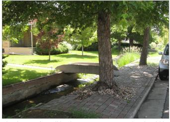
The design of small bridges spanning Bioswales should be consistent with other street and open space furnishings.
