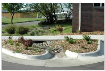
A Bulb-out containing a swale with access to street runoff
