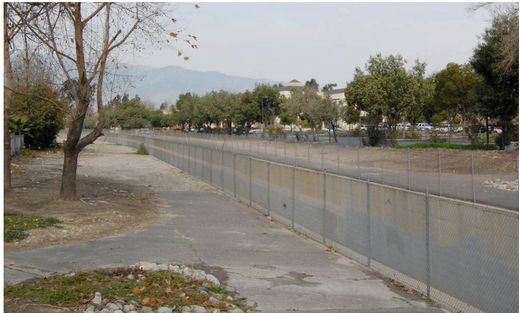
Storm drainage channel facility.
