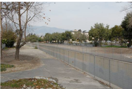
Flood Control/Utility Corridor
