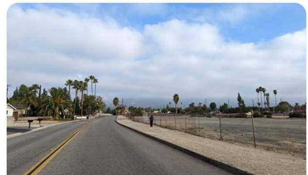
Adding sidewalks along Alta Cuesta Dr. will provide sidewalk gap closure between Base Line Rd. and Valle Vista Dr.
