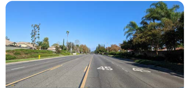
Existing roadway with 5' bike lane on 19th St.
