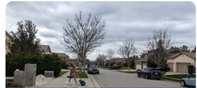
A curb ramp with tactile bumps can improve ADA access for pedestrians traveling across Stoneview Rd. to the neighborhood paseo
