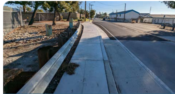
Widening sidewalk to a wider space serving bicyclists and pedestrians connecting to Cucamonga Creek trail
