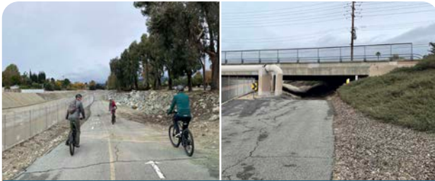
Cucamonga Creek Trail resurfacing and access enhancements would greatly improve the biking experience on the trail.
