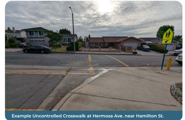
Example Uncontrolled Crosswalk at Hermosa Ave. near Hamilton St.
