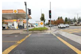
Crosswalk lacking high-visibility striping.
