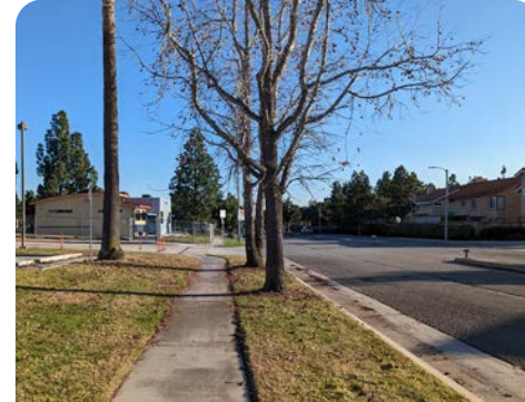
Wider sidewalks along the Terra Vista Elementary School frontage can serve bicyclists and pedestrians.
