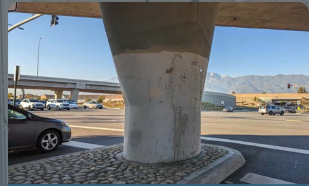
The south leg crosswalk striping at the intersection of East Ave. and I-15 can be restriped so that the highway pillar does not obstruct the crosswalk.
