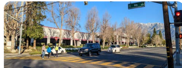
Curb ramps at Archibald Ave. and 9th St. can provide ADA access near Cucamonga Elementary school.
